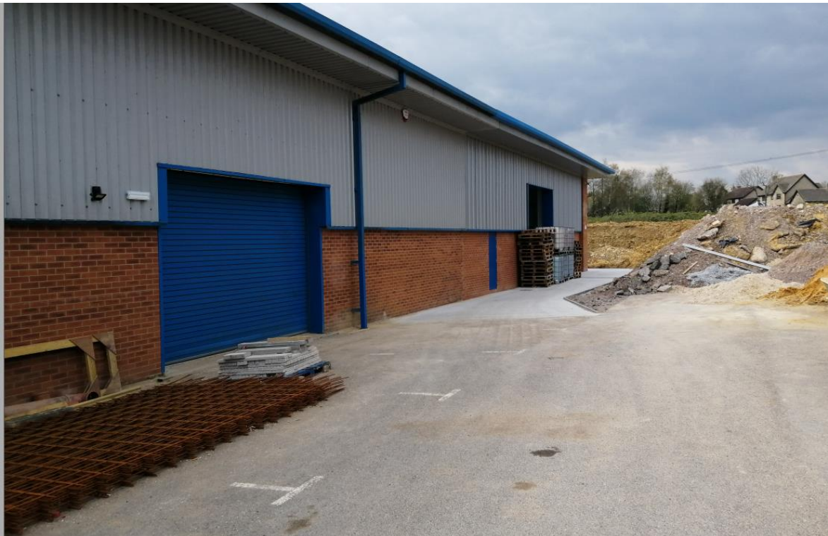
Existing goods in and our door, the extension and new goods in/out door and the bund
